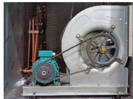
The motor is factory wired to the control panel where a dedicated contactor is located and is protected by an overload relay. The group of fan and motor is located on a rigid base which is isolated from the rest of the unit by rubber vibration isolators.
